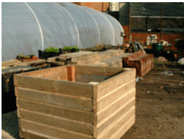
Wooden planters under construction
